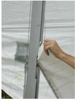
10. Attach the traveller block to the slider in the traveller track.
